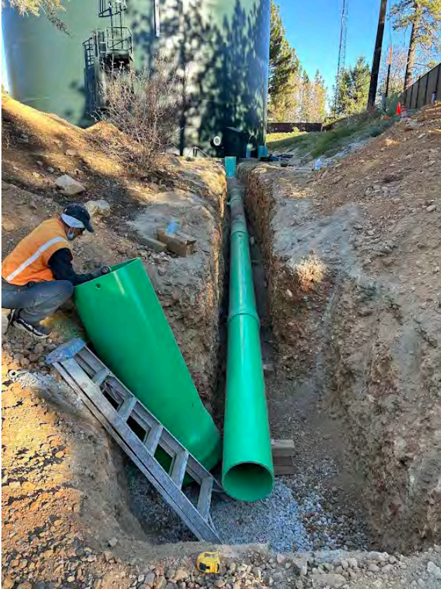
Drain Line and Catch Basin Installation
