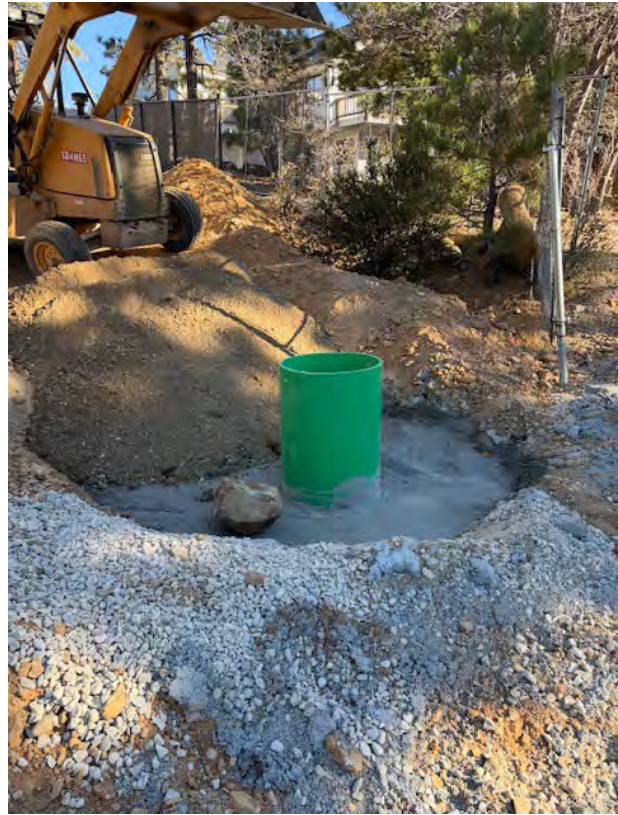
Catch Basin Installation
