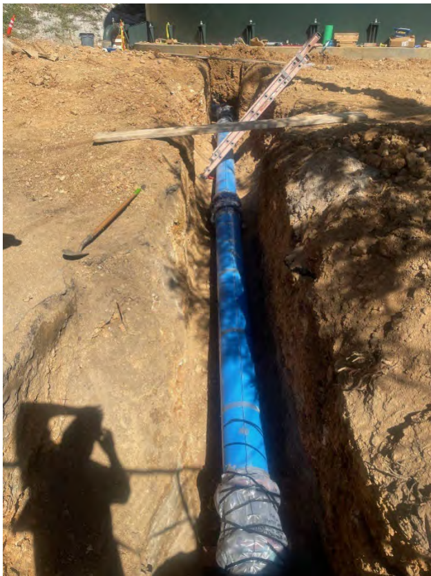
Reservoir Inlet / Outlet Line Installation
