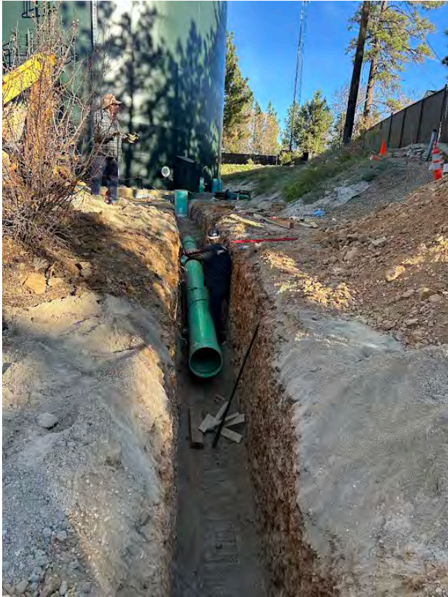
Drain Line and Catch Basin Installation
