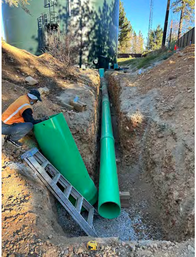
Drain Line and Catch Basin Installation
