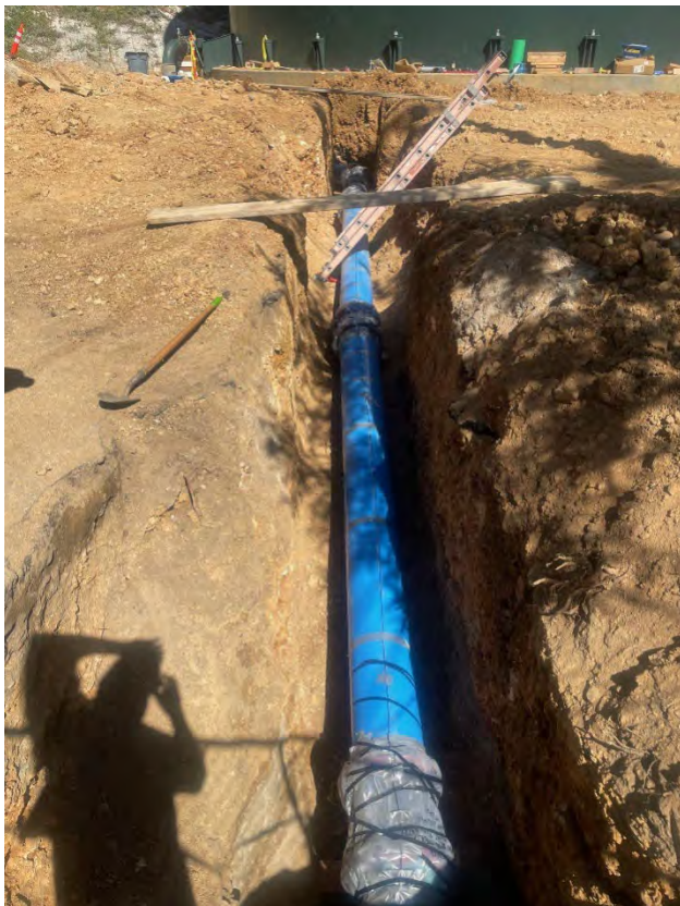
Reservoir Inlet / Outlet Line Installation
