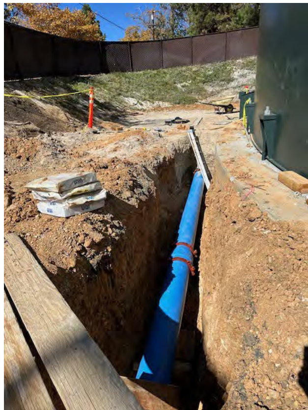
Reservoir Inlet / Outlet Line Installation
