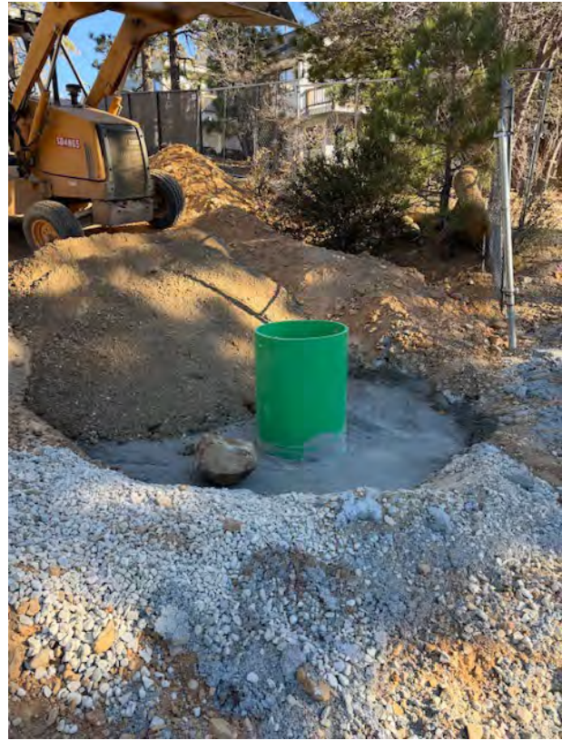
Catch Basin Installation
