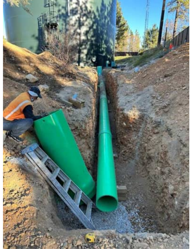
Drain Line and Catch Basin Installation
