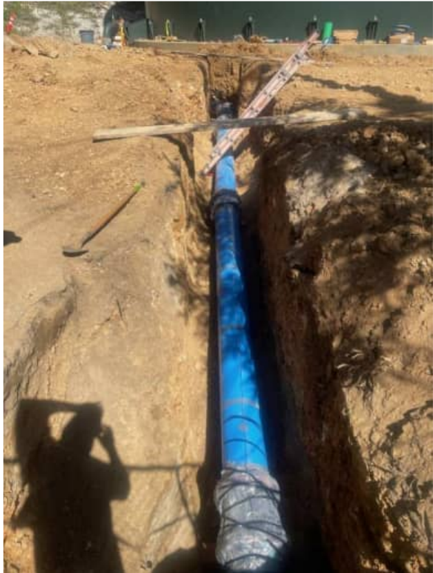
Reservoir Inlet / Outlet Line Installation
