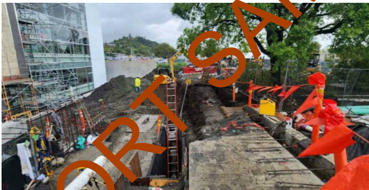
South Slope Support Shoring in-progress
