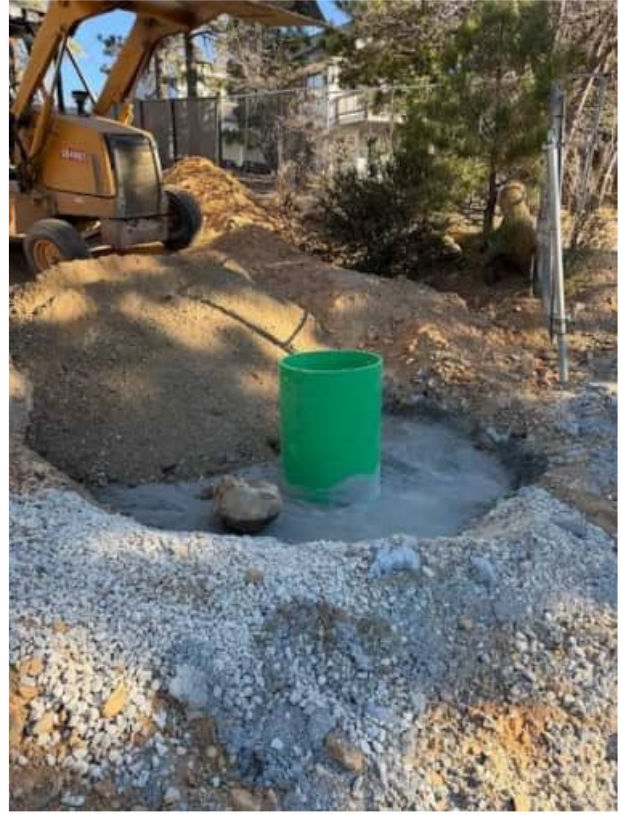
Catch Basin Installation
