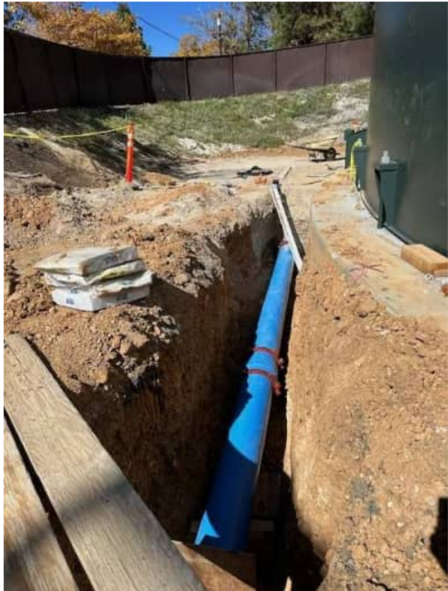
Reservoir Inlet / Outlet Line Installation
