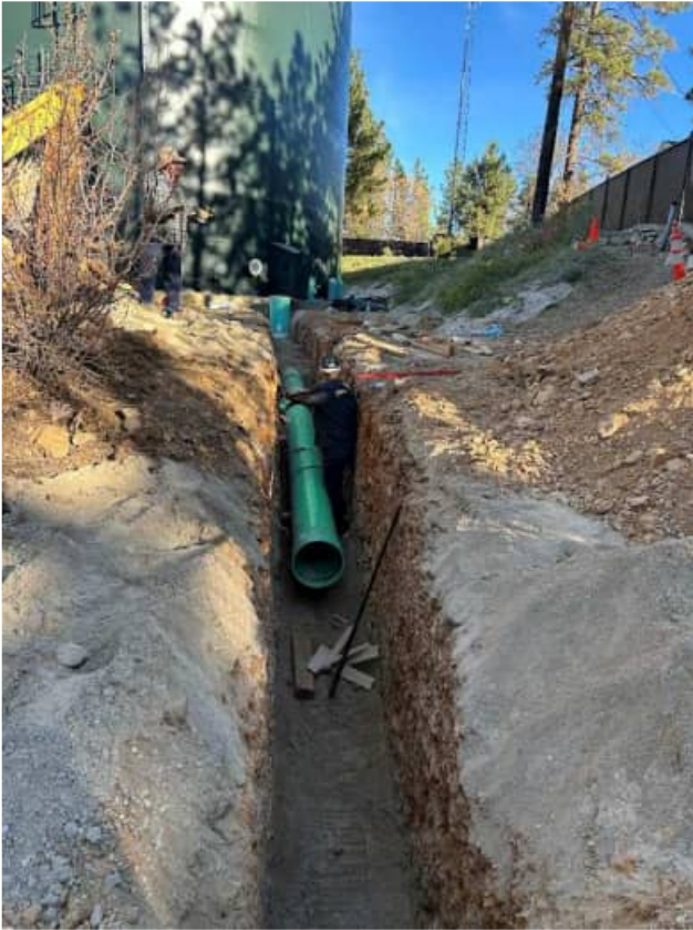
Drain Line and Catch Basin Installation
