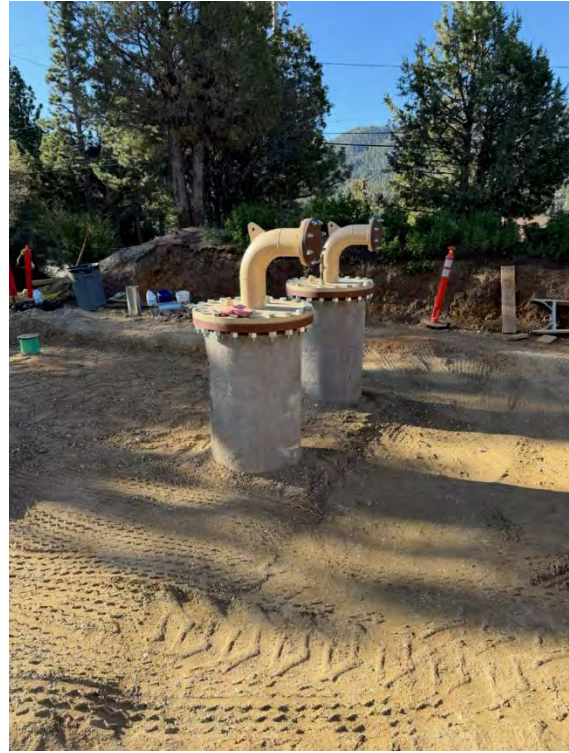
Above ground Cans and Piping after Backfill
