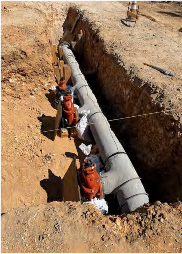
Intake Manifold Installation
