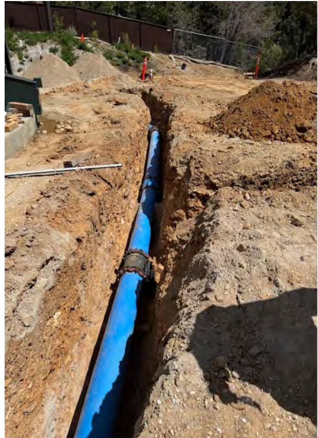
Site Piping Installation
