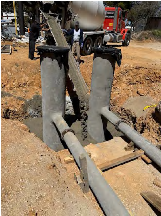
Set Pump Cans in Concrete
