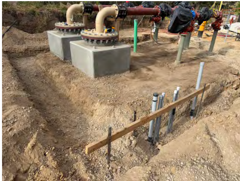
Above ground piping, footing excavation
