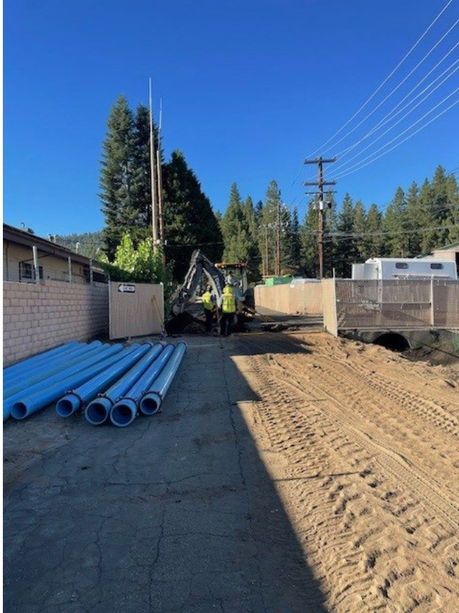
Operations Center Main, Hydrant & Service Installation
