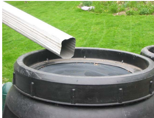
Downspout elbow used to direct water into the barrel. Can also use optional "Flex elbow" to direct the water from the downspout.
