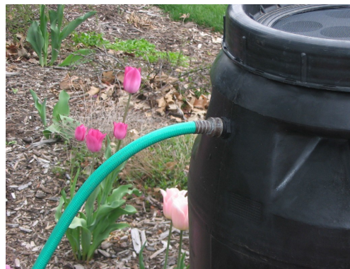
Attach garden hose to overflow fitting and direct away from the house.
